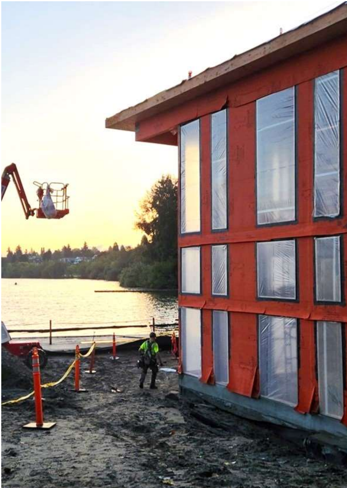
GREEN LAKE SMALL CRAFT CENTER, CONSTRUCTION 2023
